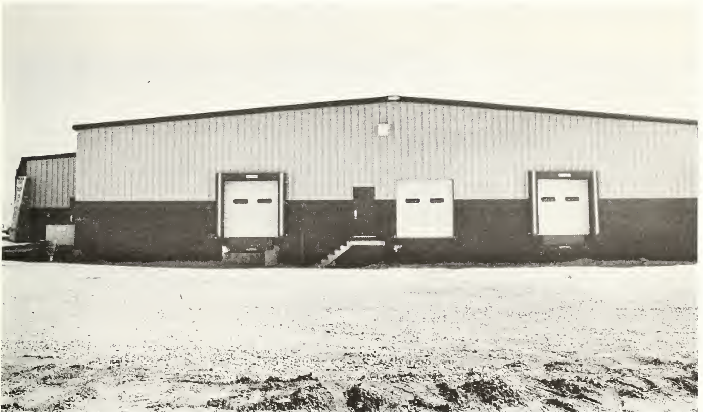
Figure 8.—Three shipping doors, two with seals, at the new plant.
