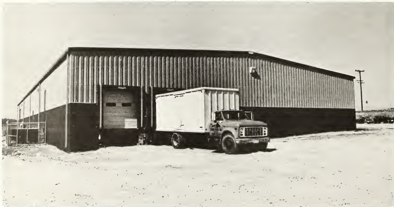
Figure 9.—Receiving doors at the new plant.
