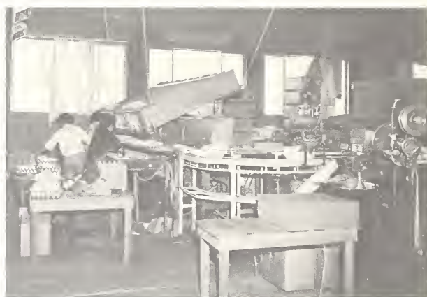
FIGURE 35.—A table for bundles of cases at makeup machine reduces labor
