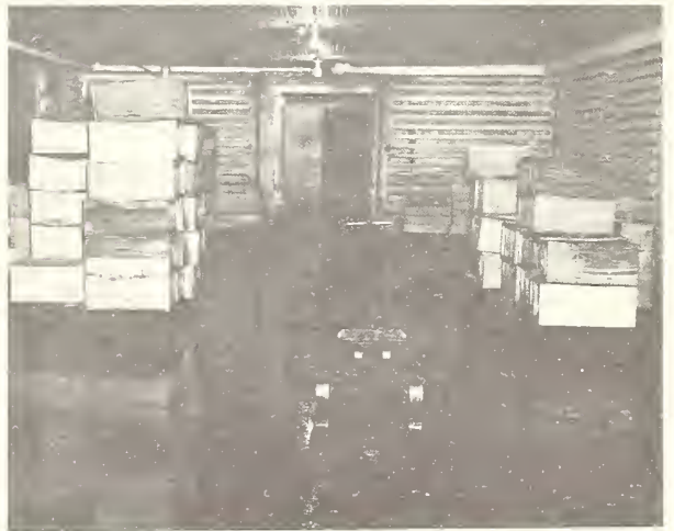
FIGURE 7.—Standing water drained from icepacked poultry was a nuisance common to coolers, work areas, and worker passageways.
