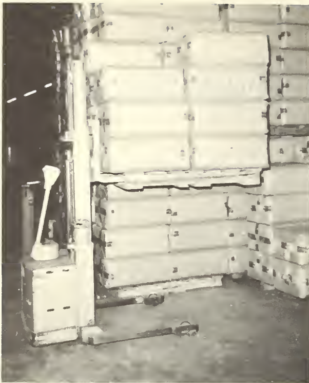
FIGURE 32.—A straddle-type electric high-lift pallet transporter high stacking a pallet load of packing materials.
