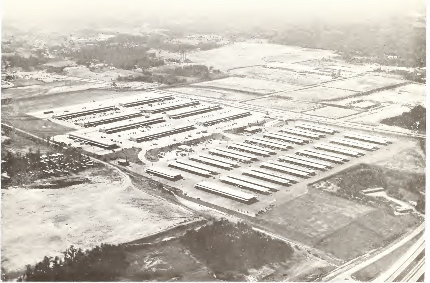
FIGURE 1.—Aerial view of a modern food distribution center.
