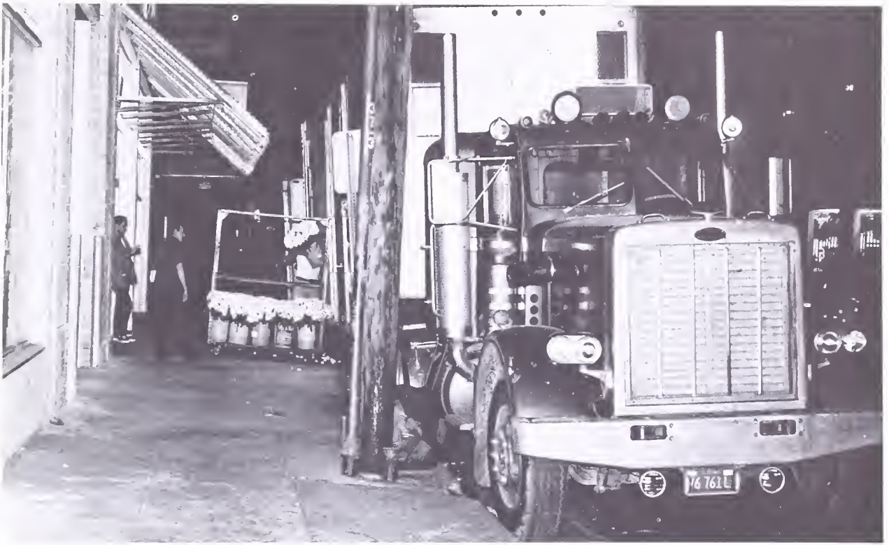
FIGURE 5.—Semitrailer being unloaded while parked parallel to curb.
