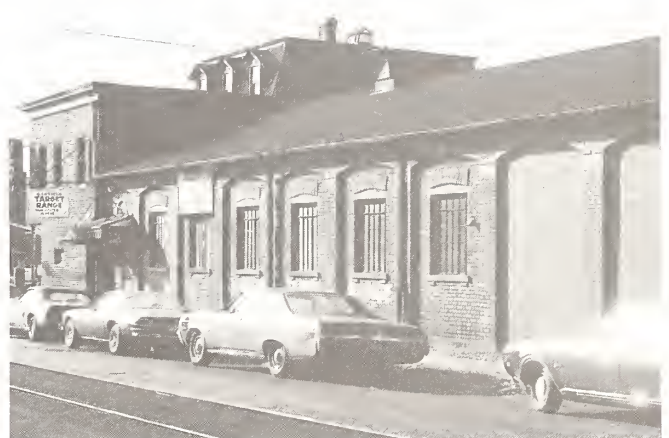
Figure 9.—Food warehouse building adapted from other use.
