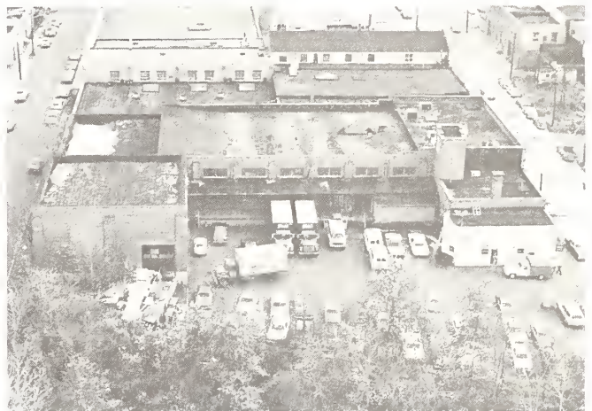
Figure 8.—Wholesale food distribution facility of obsolete design.
