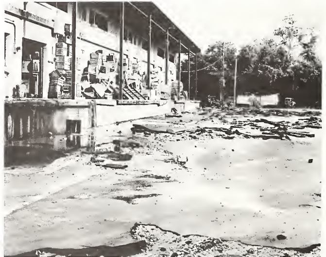
Figure 10.—Heavy flood damage on the Raleigh State Farmer's Market.
