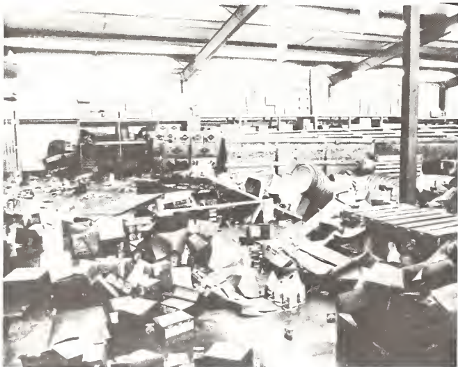
Figure 9.—Flood-damaged inventory and buildings on the Raleigh State Farmer's Market.
