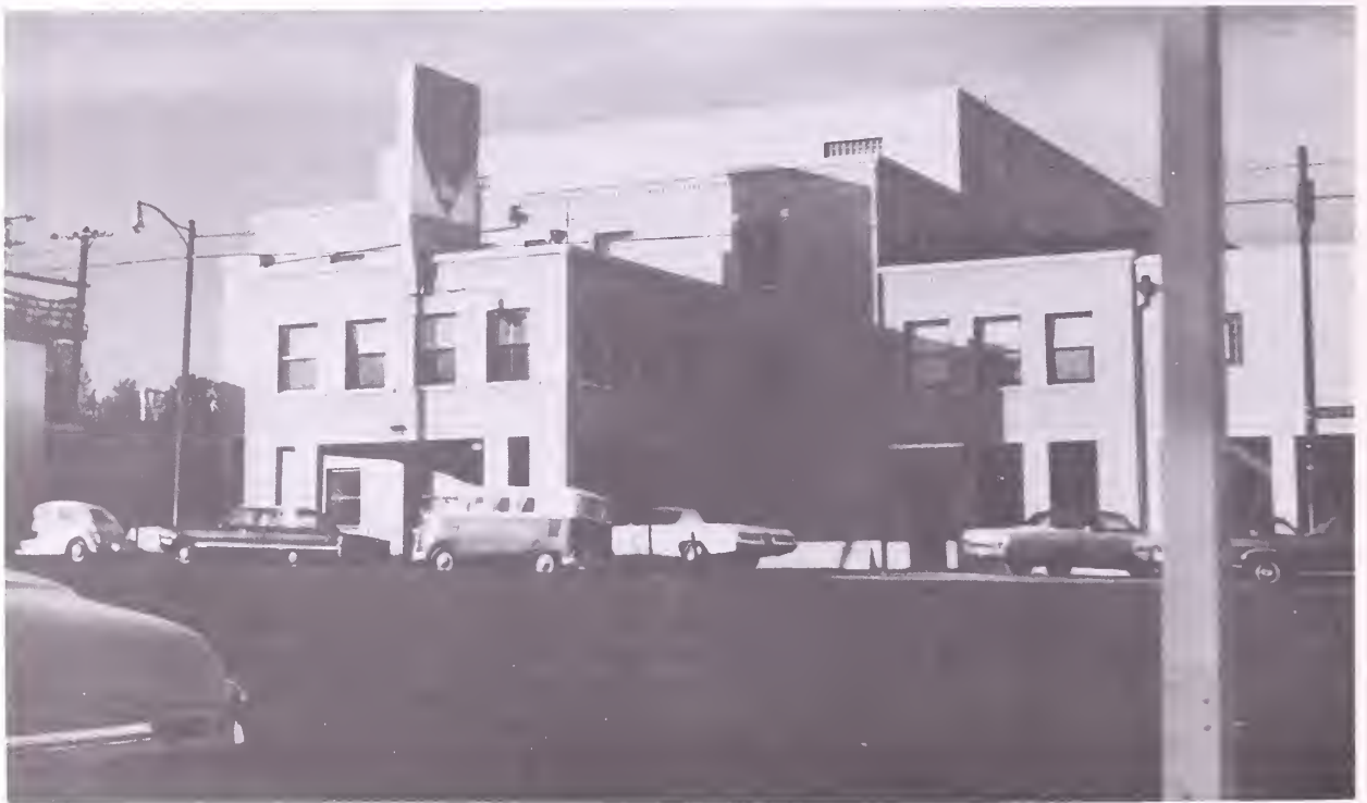
FIGURE 9.—Multistory dairy products plant.
