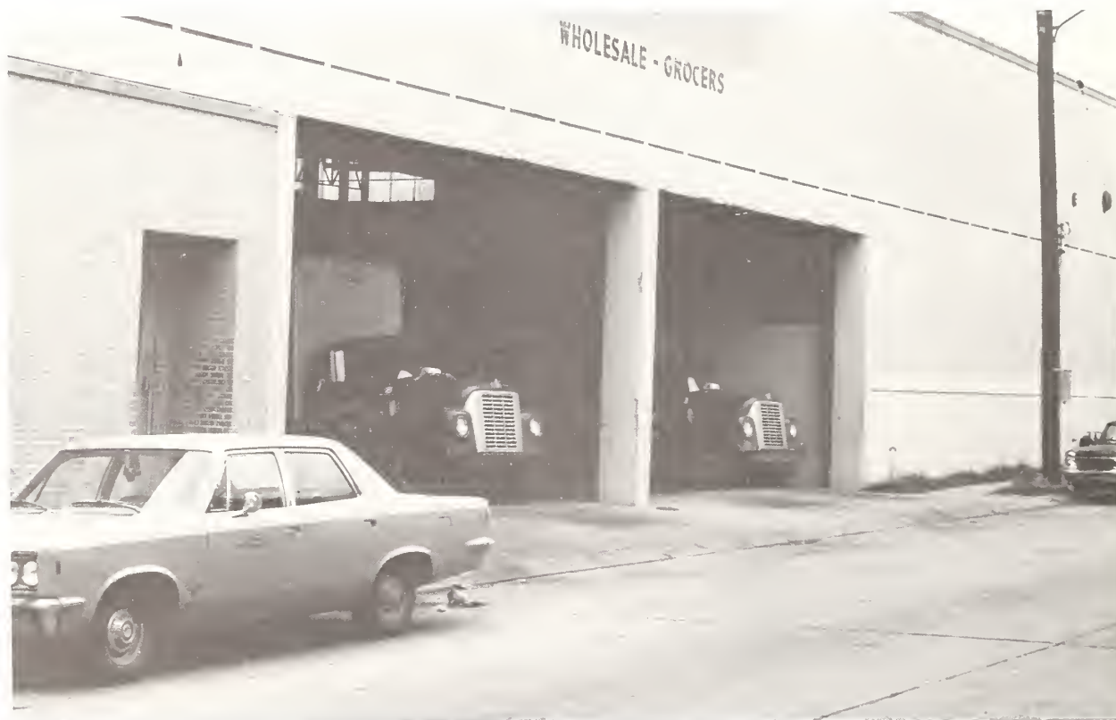
FIGURE 7.— Grocery wholesale facility with interior truck loading.
