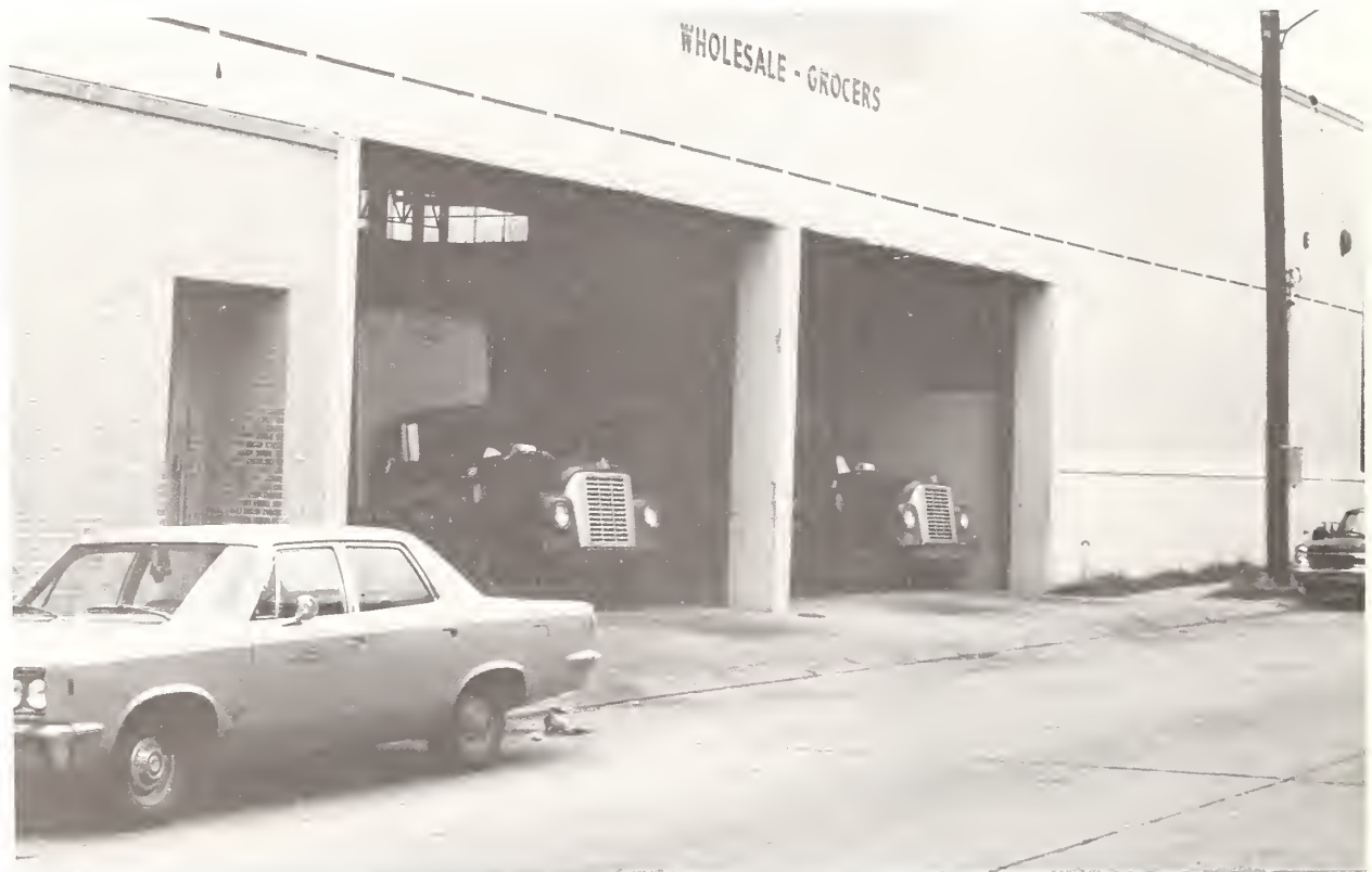
FIGURE 7.— Grocery wholesale facility with interior truck loading.
