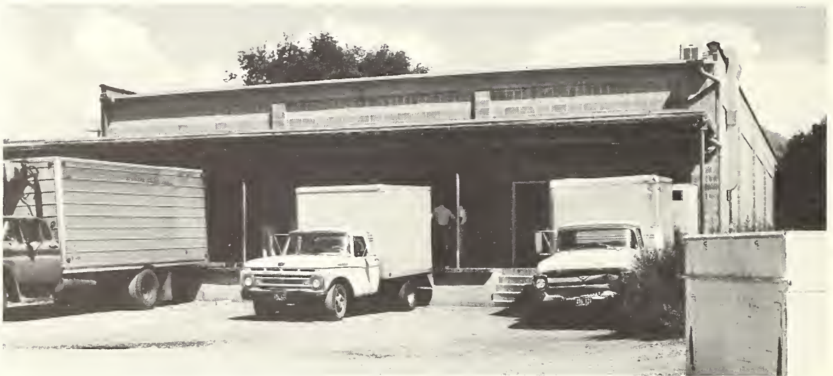
FIGURE 11.—A modern dairy products and egg facility serving the Salt Lake City area.
