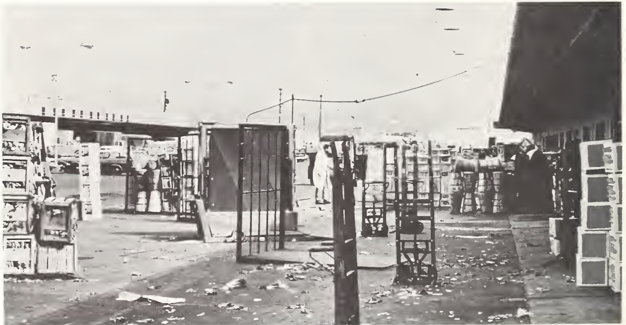
FIGURE 16.--Receiving area at ground level.
