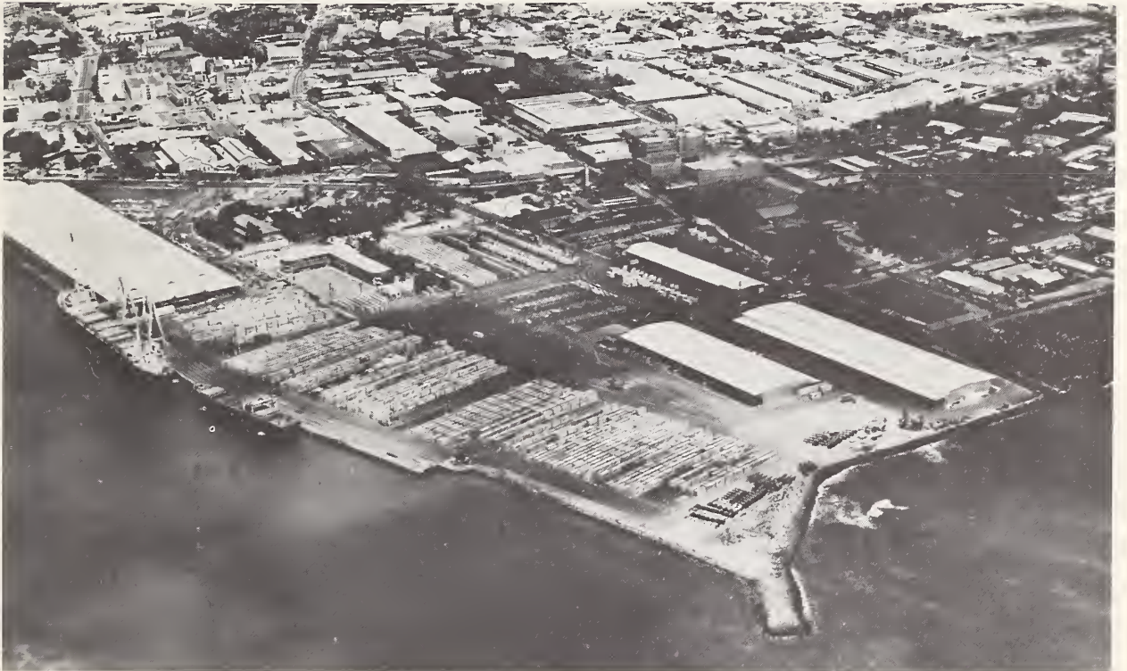
FIGURE 3.--Aerial view of pier 2 and container yard.
