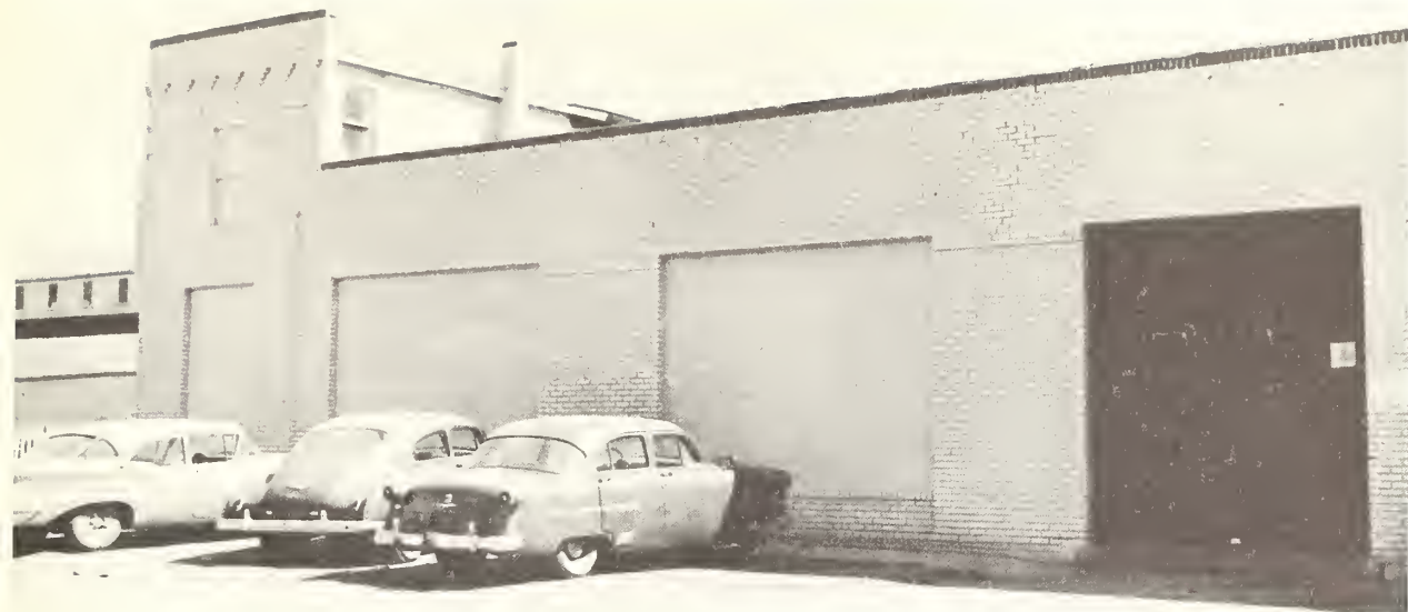
Figure 6.—Street-level receiving and shipping area at plant C increases handling cost.
