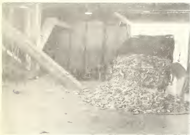
Figure 18.—This small unloading pit is a bottleneck.
