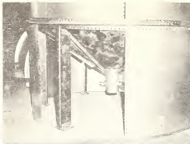
Figure 12.—Conical steel hopper bottom.
