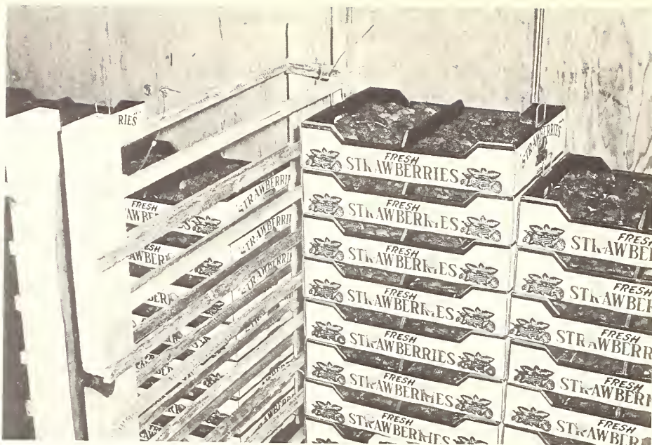
Figure 14. --Method of loading container B in express car. Lengthwise gate is used to take up crosswise slack.
