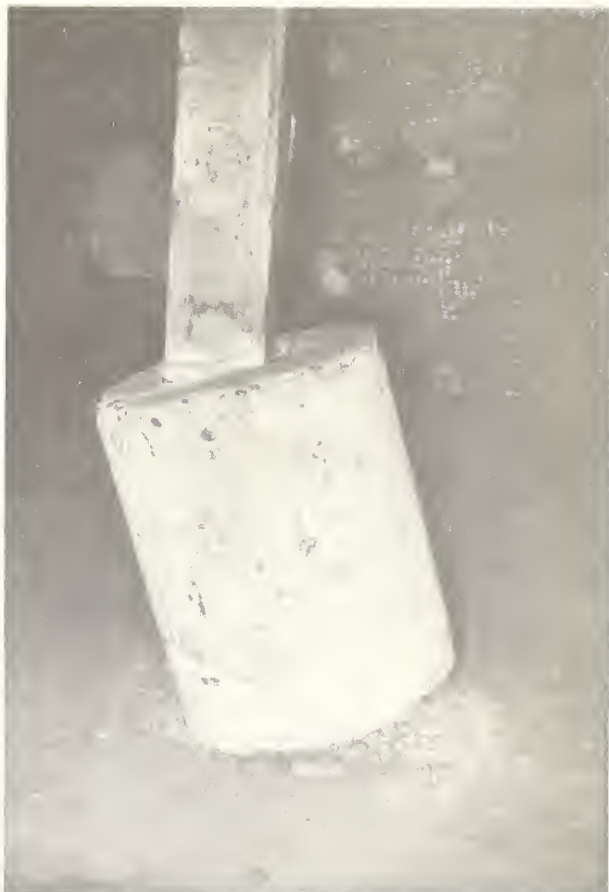
FIGURE 5.—Column and improperly constructed concrete column guard damaged by clamp trucks.
