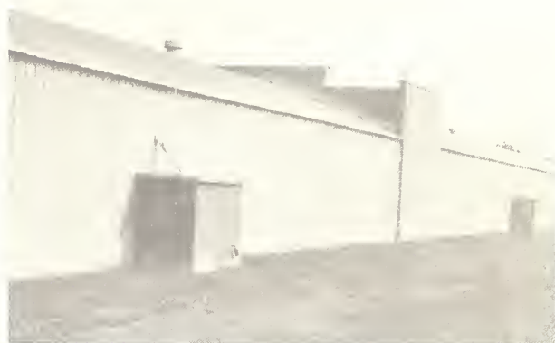
FIGURE 13.—Masonry firewall separating two compartments.
