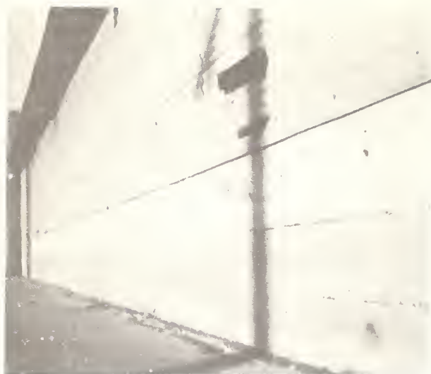
FIGURE 21.—Concrete wall base, 4 feet high, prevents clamp-truck damage to wall.
