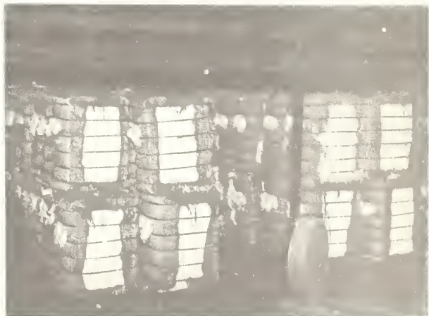
FIGURE 6.—Structural framing and sprinkler pipes limit stacking of bales to 2 high on head.
