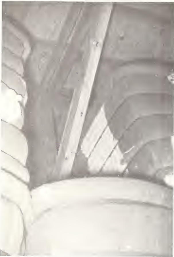
FIGURE 7.—Column knee braces using bale storage space.
