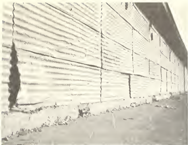
FIGURE 3.—Wall damaged by clamp trucks.
