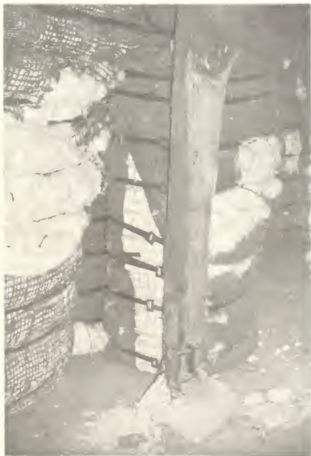
FIGURE 4.—Column damaged by clamp trucks.
