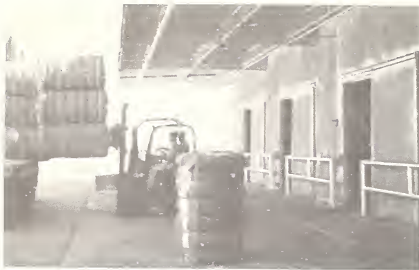
FIGURE 16.—Door and walls in truck receiving area protected from clamp-truck damage by 4-inch steel pipe.
