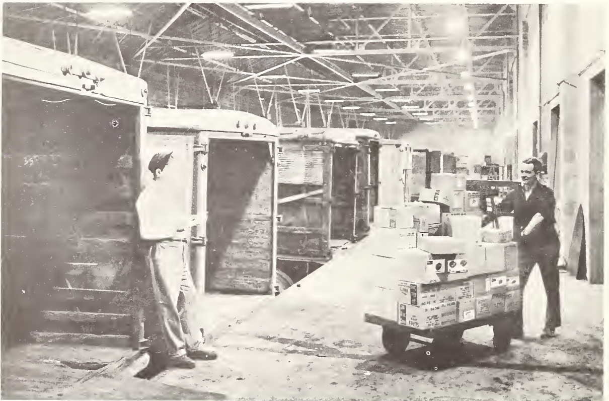
Figure 9.--Wall-mounted flood lamps used to light the interior of delivery trucks.
