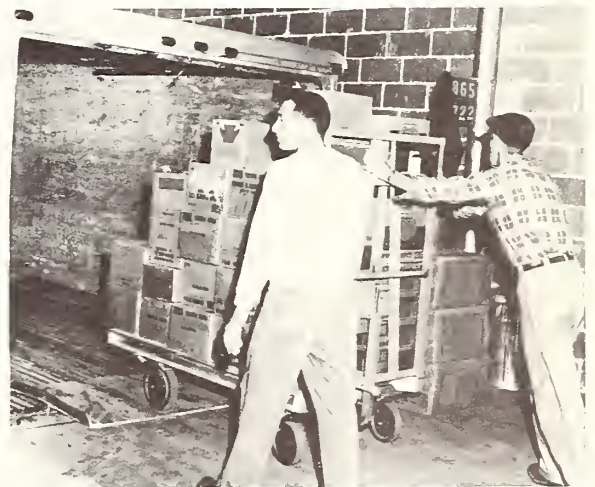
Figure 5.--A delivery trailer at a dock built at the proper level.
