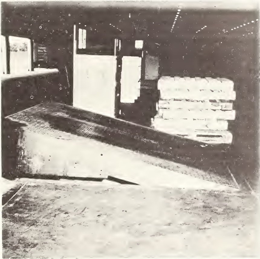
Figure 19.--A dock that automatically adjusts to different truckbed heights.
