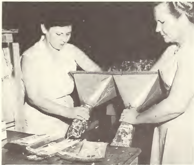
Figure 11.--Cellophane bags being filled with tossed salad through a funnel-like chute
