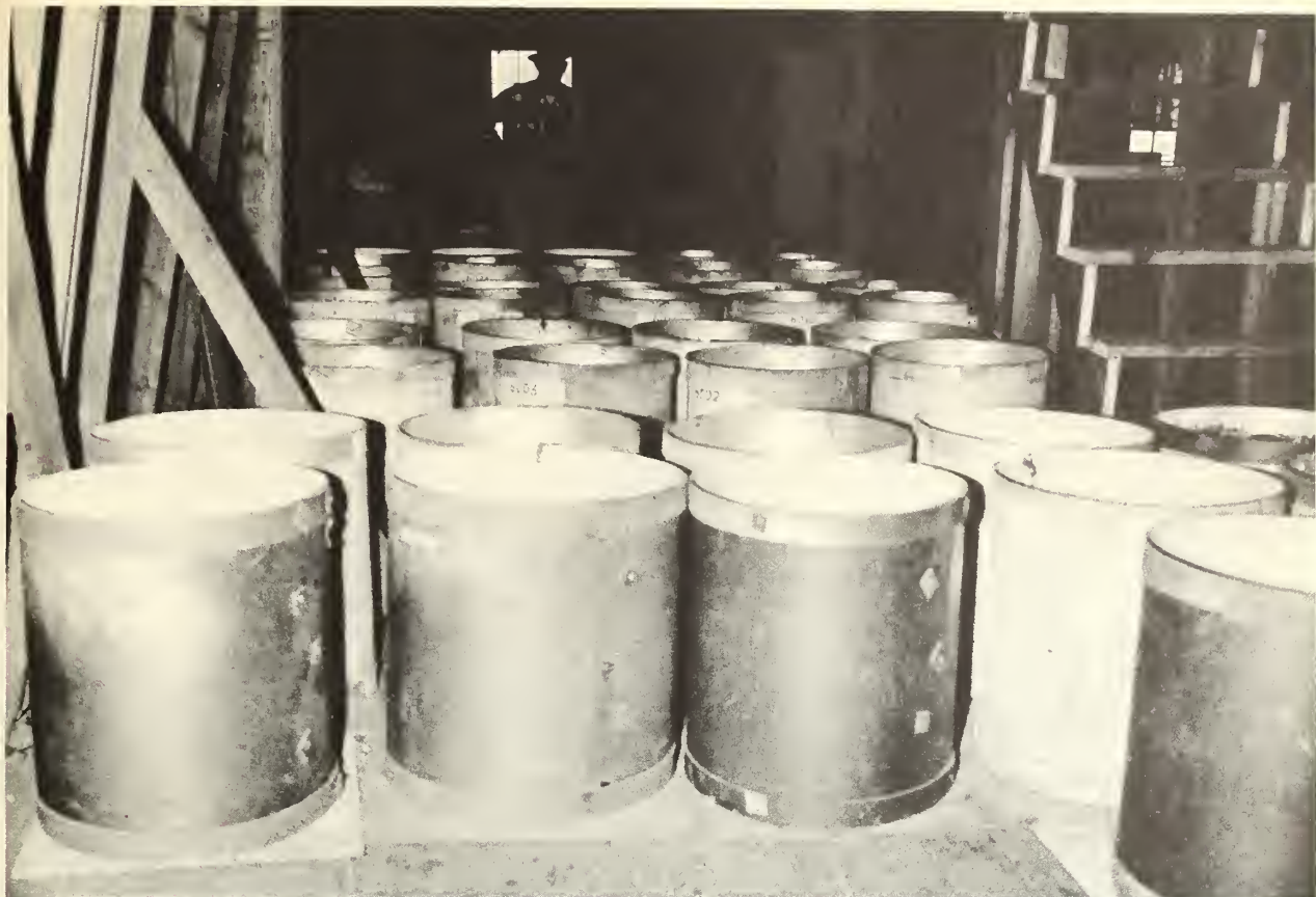
Figure 1. --View of drum-type small bins arranged in random pattern in unheated barn.
