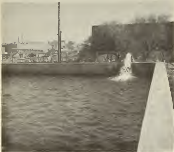
Figure 21.—The Stockyards water reservoir.
