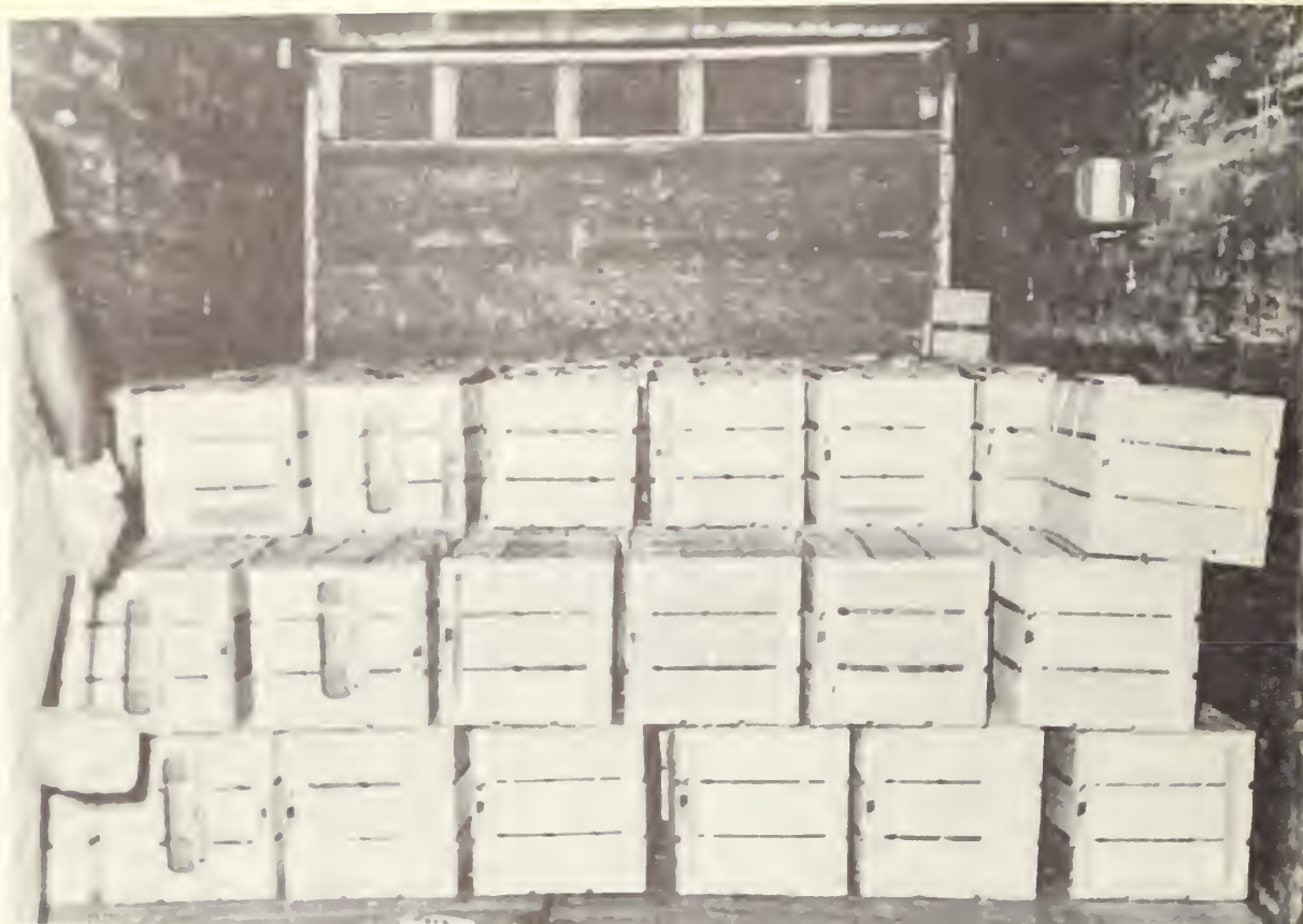
Figure 10.--Cross-section of a refrigerator carload of 60-pound wirebound crates at the shipping point.
