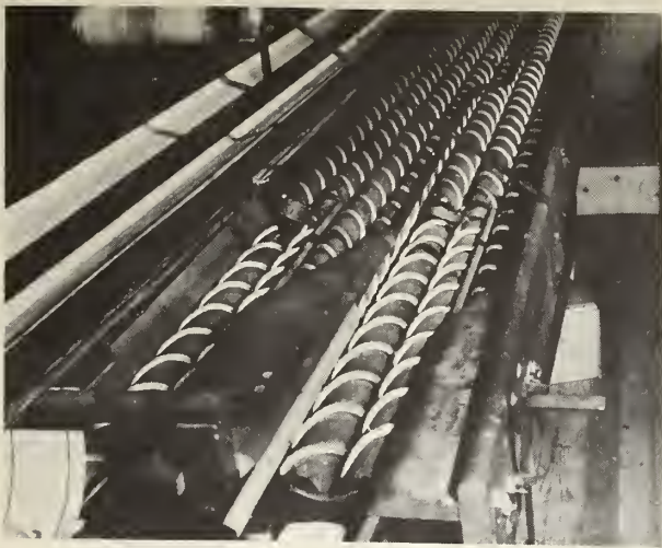
FIGURE 2.—A spiral-roll sorting table.
