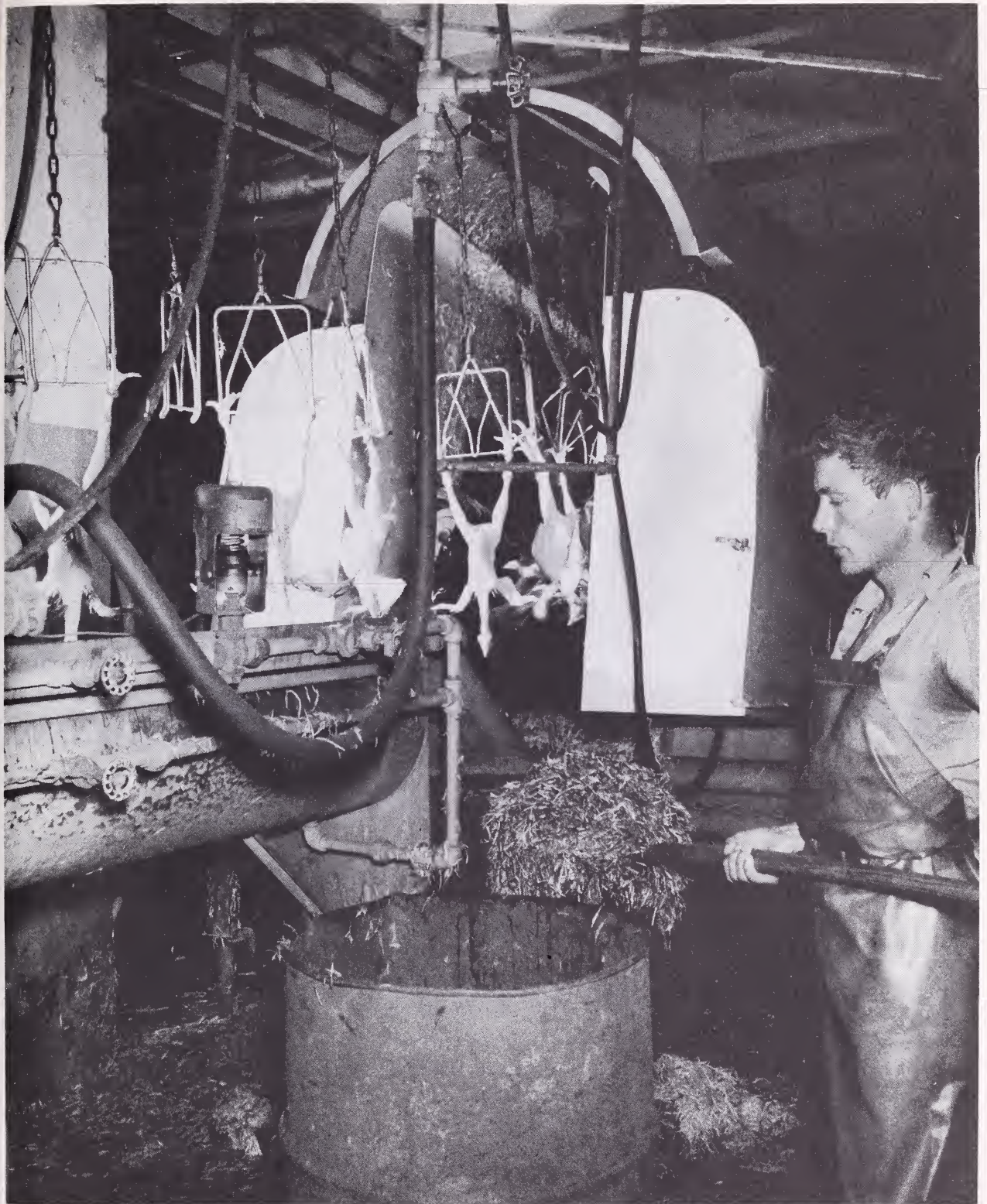
Figure 3.--Collecting feathers from picking machine area.
