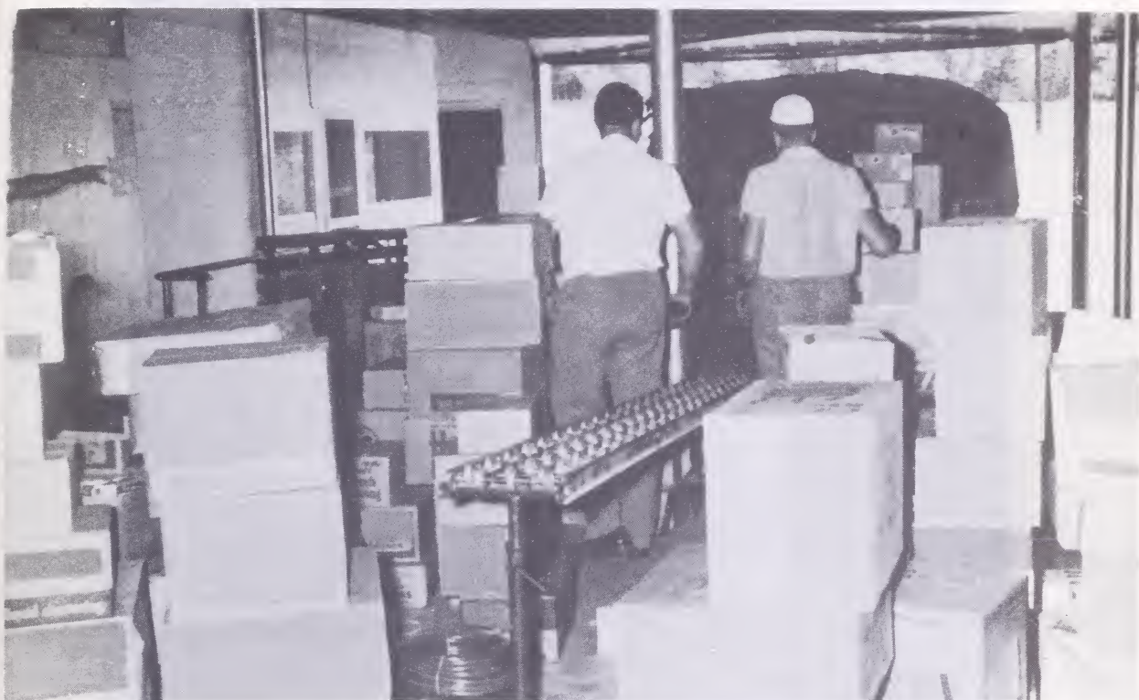
Figure 11.--A short conveyor line used to reassemble merchandise into individual retailer orders and load it in a delivery truck.
