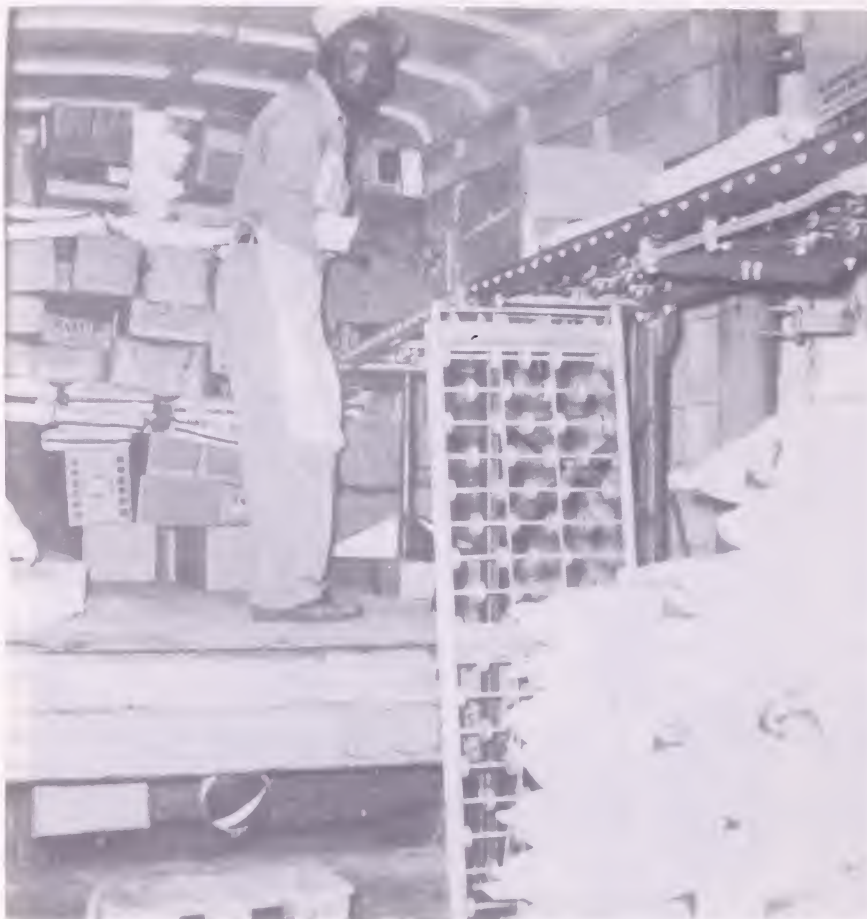
Figure 15.--Merchandise placed on the conveyor in the selection area is being loaded in the truck from the same conveyor.
