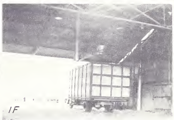
Figure 1.--Views of three storage facilities in California. (1-A and 1-B) Two of three concrete houses with central unloading suction. (1-C and 1-D) Three all-steel houses, with gin in middle and unloading suction on house adjacent to second gin. (1-E and 1-F) Movable-rack system under shed built in U-shape and one rack on truck, equipped with hydraulic lift, at unloading suction, preparatory to being moved to shed.
