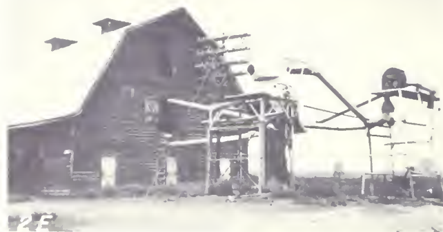
Figure 2.--Three storage facilities in Yazoo-Mississippi Delta. (2-A and 2-B) One side of concrete-block house with unloading suction in cleaning annex adjacent to storage house. (2-C and 2-D) Four wooden houses with unloading suction. (2-E) Typical plantation barn loft used for storage, with unloading and loading suction. Not shown is tractor which supplies power.
