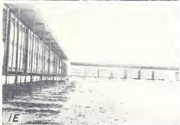
Figure 1.--Views of three storage facilities in California. (1-A and 1-B) Two of three concrete houses with central unloading suction. (1-C and 1-D) Three all-steel houses, with gin in middle and unloading suction on house adjacent to second gin. (1-E and 1-F) Movable-rack system under shed built in U-shape and one rack on truck, equipped with hydraulic lift, at unloading suction, preparatory to being moved to shed.
