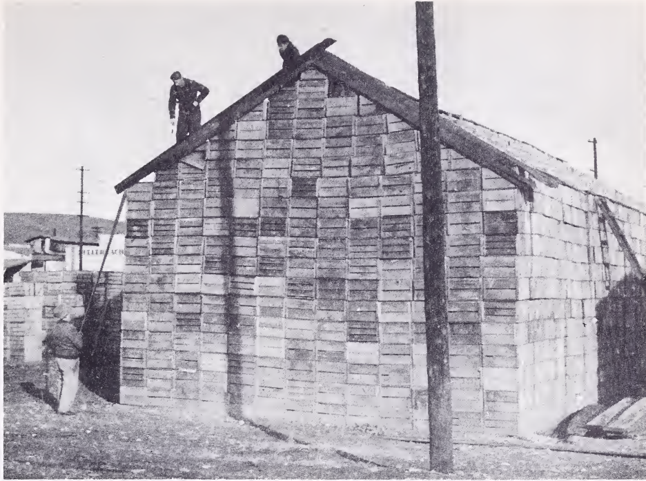
Figure 9.--Workers removing the roof from a box house.
