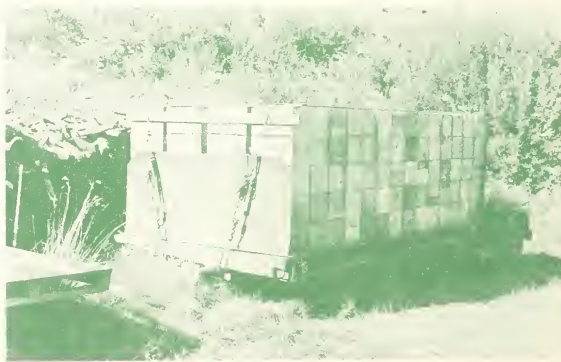
FIGURE 23. --Loaded road truck with wide bridge plate used in method H.
