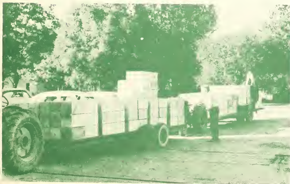
FIGURE 3. --Trailers with lengthwise loads.
