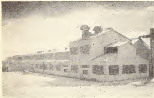
FIGURE 2.—Mill building of cottonseed oil plant.
