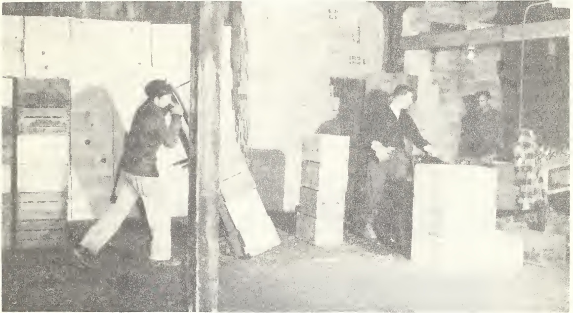
Figure 87.--A hand trucker supplies a dumper from a temporary bank.
