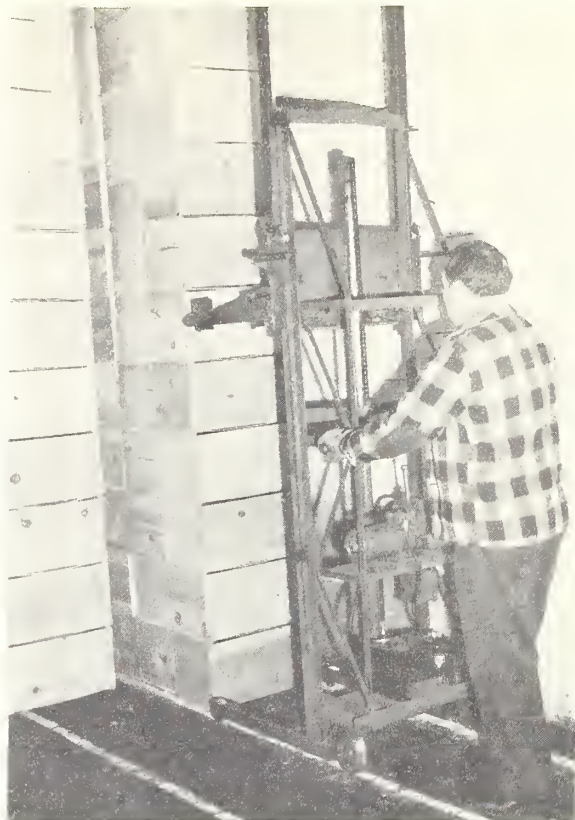
Figure 39.--After the top stacks are lowered the worker withdraws the machine from the stacks and the clamping arms are lowered for another pick up.
