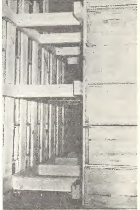
Figure 113.--An approved type of car brace (Type B) with the main support vertical.
