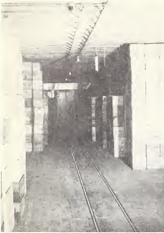
Figure 7.--Floor chain conveyor in a cold storage room.
