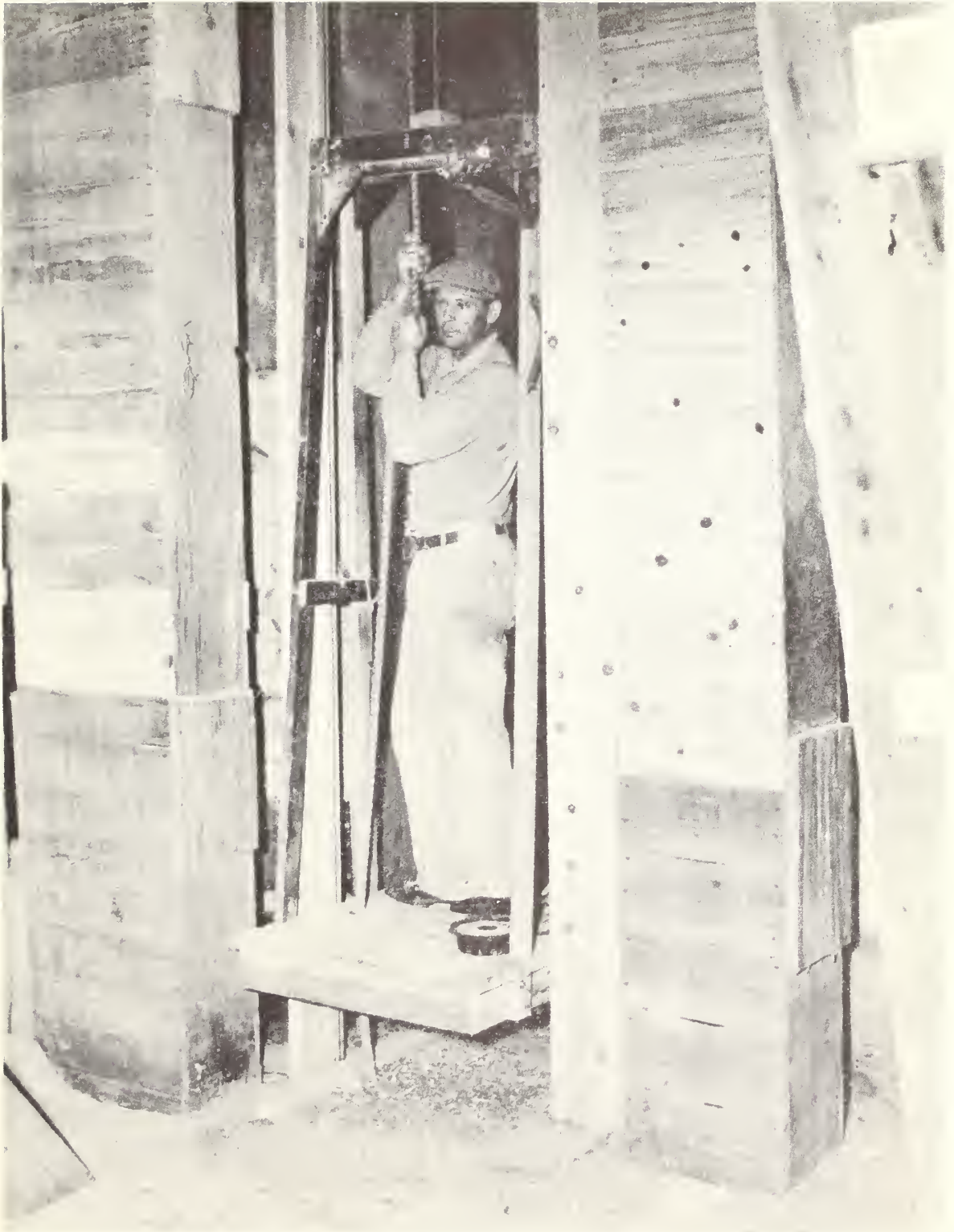
Figure 21.--Elevator legs of wooden construction are spaced to permit placement of manlift between them.
