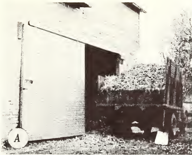
Figure 10.--A, For many years this cob bin was located at ground level. A scoop and man labor loaded the trucks with cobs for disposal outside city limits. B, Later, a cob bin was built, allowing trucks to back in and load direct from the bin. Costs of operation were reduced, but a cob incinerator would further decrease costs when cobs and other wastes are not used as feed for livestock.
