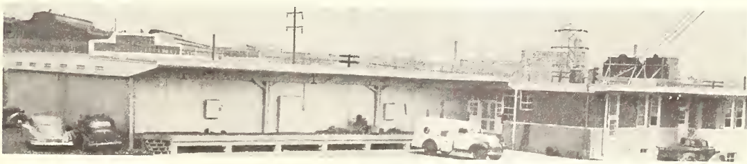
Figure 1.--A private frozen food warehouse and plant. A common platform is used for in-and-out truck movements. This plant is of prefabricated construction. Rail connections, although not presently needed, are available for possible future use.
