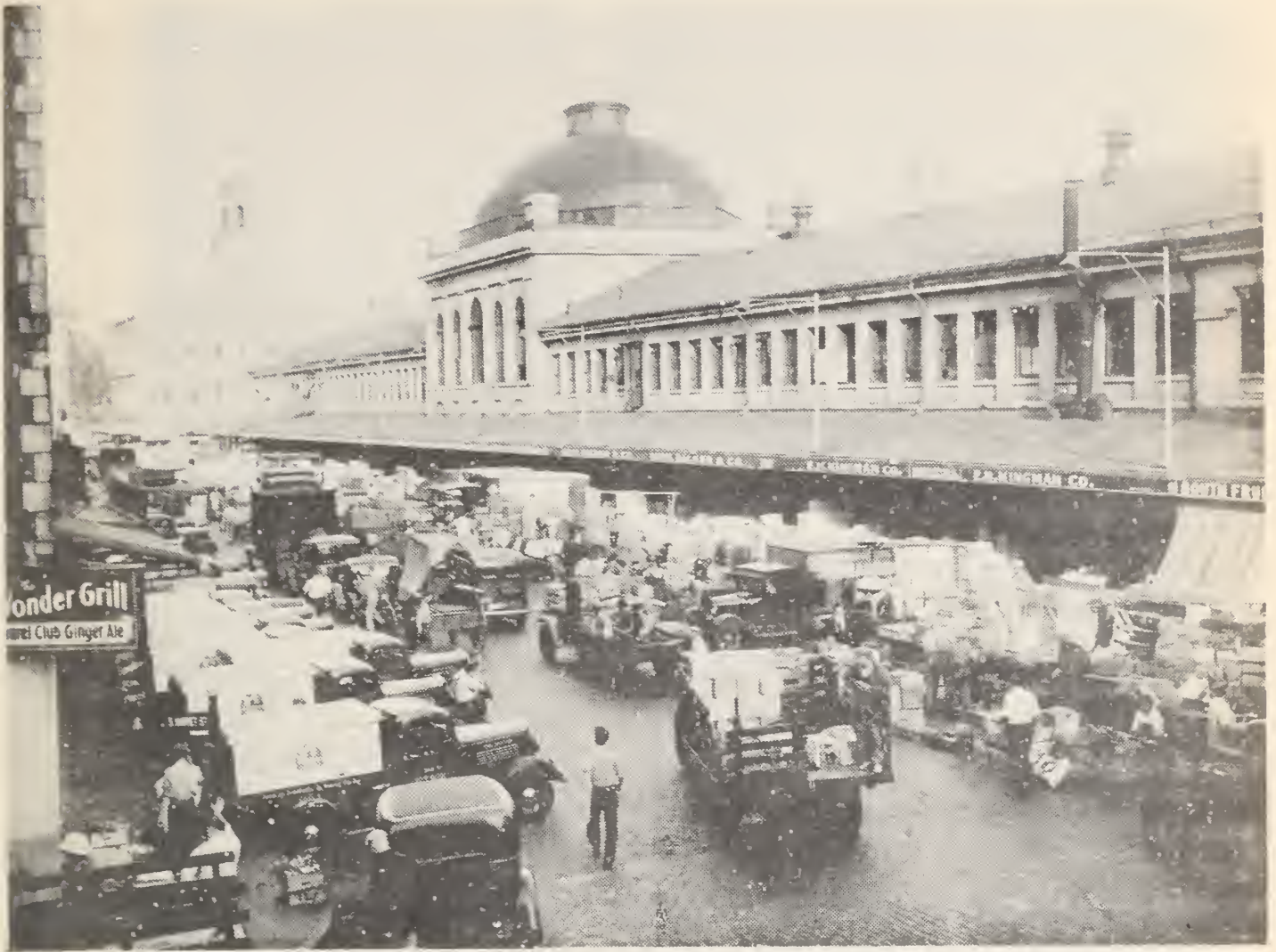
Figure 4. - Faneuil Hall Market, Boston, Mass. One of the oldest and most famous farmers' markets in the United States. This market was built in 1740 and the one preceding it was established in 1634. The space originally provided in the open streets for selling by growers is now entirely inadequate.
