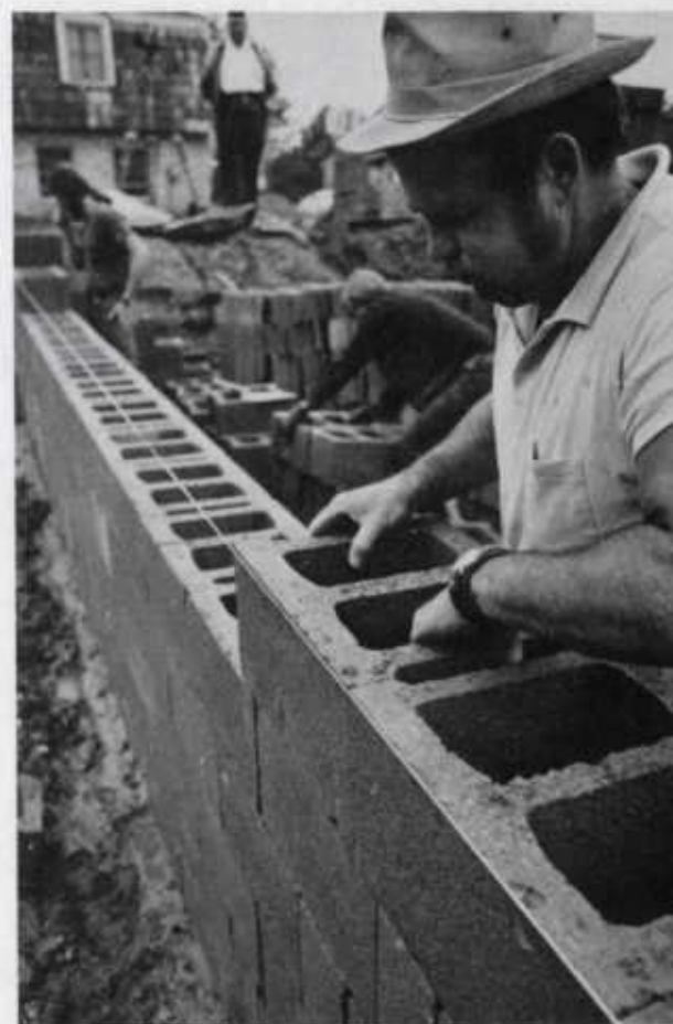
Figure 8.—Mason's line held between corners with wooden hooks. Lay wall without mortar to line.
