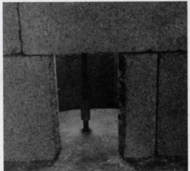
Figure 18.—Attach connector end of rod to the tie-down bolt set into the concrete footing or floor slab.
