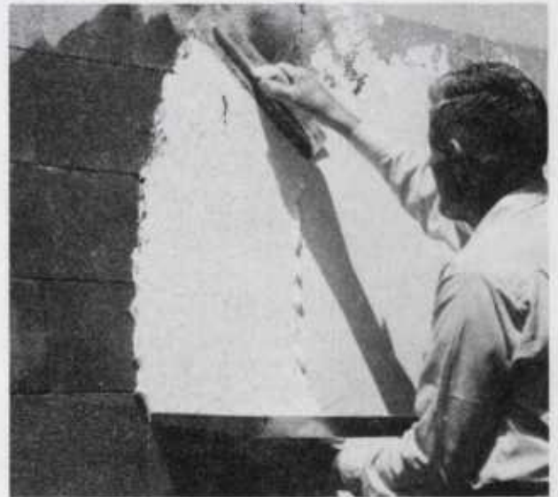
Figure 23.—Work the bonding mix from a hawk onto the wall with a plasterer's trowel. Note the specially made hawk with turned-up edges on three sides to prevent spilling the relatively thin mix.
