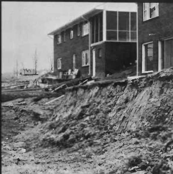
Figure 5.—Unstable soil like this, which shrinks when dry and swells when wet, has a high clay content in the upper 3 to 4 feet. To check, press a small sample of the moist soil between the thumb and index finger. If it is clay, a ribbon forms. Such soil is fine textured, sticky when wet, commonly dark, and feels like putty. When dry, clay soil may have many cracks 2 to 4 inches wide and 10 to 20 inches deep. The surface may be sandy, silty, or clayey, underlain by dense plastic clay.
