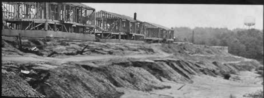
Figure 16.—To build on hillsides requires additional excavation for a solid foundation. Except for extremely steep slopes, however, runoff and erosion can be controlled with proper soil and water conservation practices. On most slopes that have clayey soil it is difficult to establish a good cover of grass and trees.
