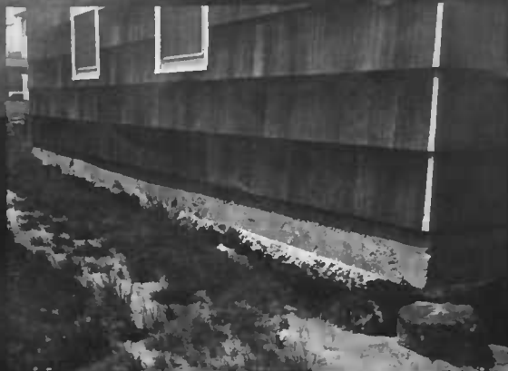
Figure 8.—More than 20 houses costing about $20,000 each were built in a former swamp area with highly organic soil. The swamp had been drained, fill added, and a cement slab placed on deep piling. In 2 years, the soil around these houses had settled about 2 feet. The soil will continue to settle at about this rate for years to come. This problem is difficult and costly to correct.
