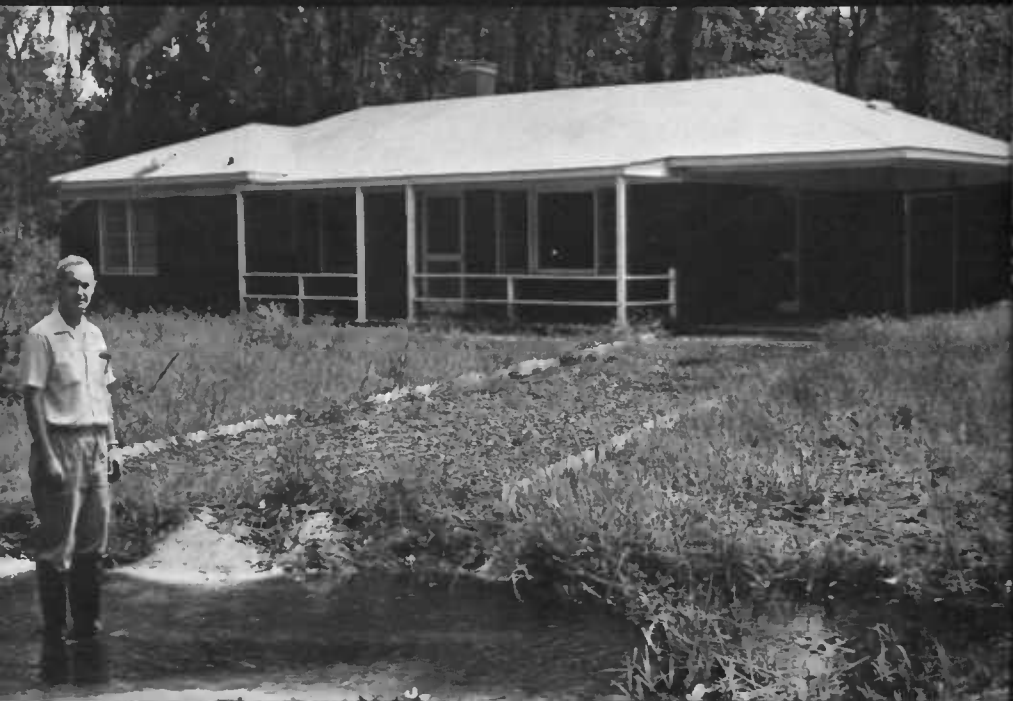
Figure 14.—Soil with a permanent or seasonal high water table causes problems for on-site sewage disposal, for underground utilities, and for basements. A high water table usually means special building foundations for stability.
