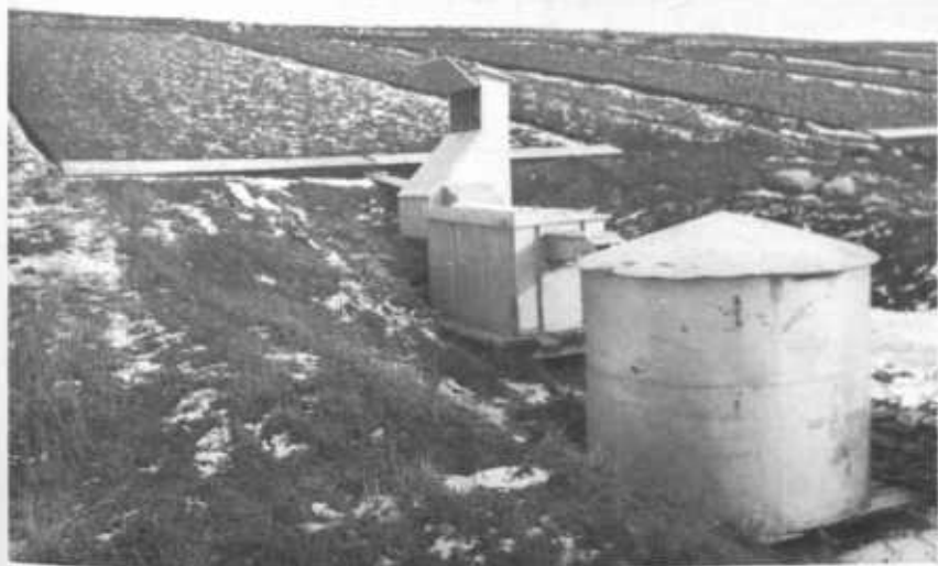
FIGURE 2.—A typical installation to measure runoff from plots at Marcellus, N.Y.
