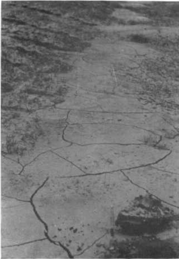
Figure 2.—Silt deposition in the channel of a basin terrace caused by erosion of the cut slope above.
