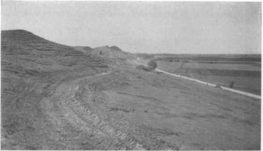
Figure 4.—Basin terraces protect more nearly level areas from runoff water from steep areas above.
