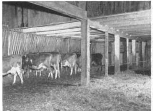
FIGURE 22.—Feeding arrangements in existing buildings may be satisfactory for loose housing. Electric fence separates feeding and resting areas in this barn.
