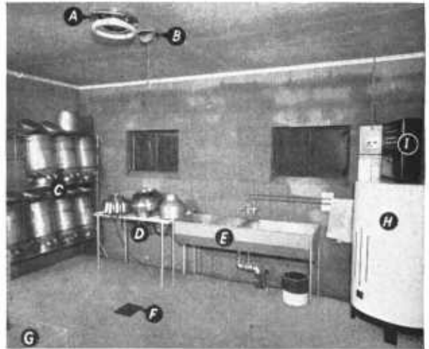
FIGURE 10.—Milkhouse interior showing fluorescent light (A), ventilator (B), can rack (C), drying table (D), wash vats (E), floor drain (F), corner of cooler (G), water heater (H), and space heater (I).
