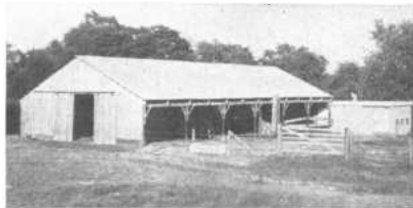
FIGURE 25.—This well-arranged loose-housing system includes a milking room and milkhouse located at the far right. It meets local requirements for Grade A milk production.
