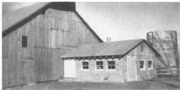
FIGURE 24.—An inexpensive milking plant attached to an existing barn will satisfy requirements for Grade A milk production in many areas.
