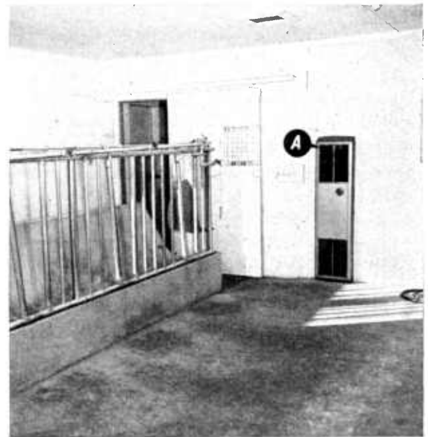
FIGURE 9.—Interior of a milking barn without stall partitions or gutter. A heater (A) has been installed on the back wall.
