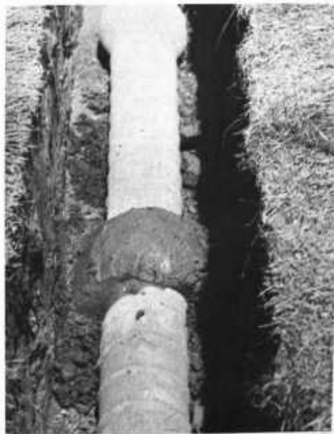
FIGURE 5.—Mortar joint in concrete sewer pipe showing mortar band used for additional protection against root entry. (Photo courtesy Portland Cement Association.)
