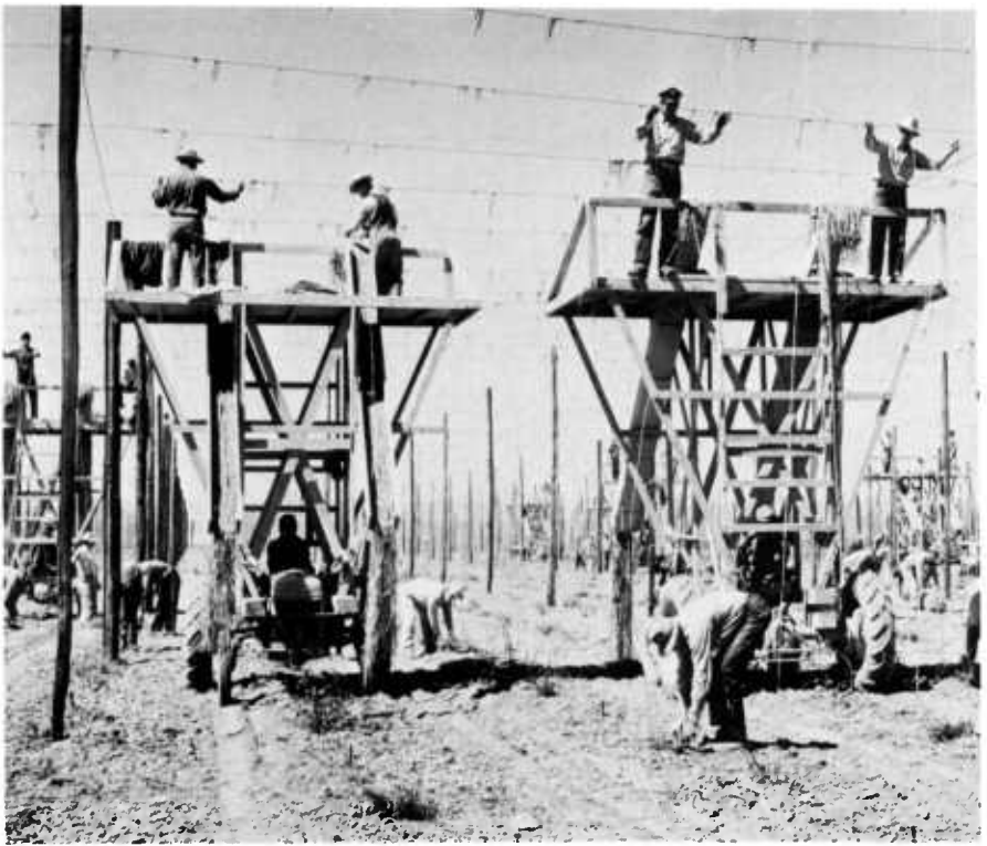
FIGURE 12.—Stringing crews at work showing use of high carts.
