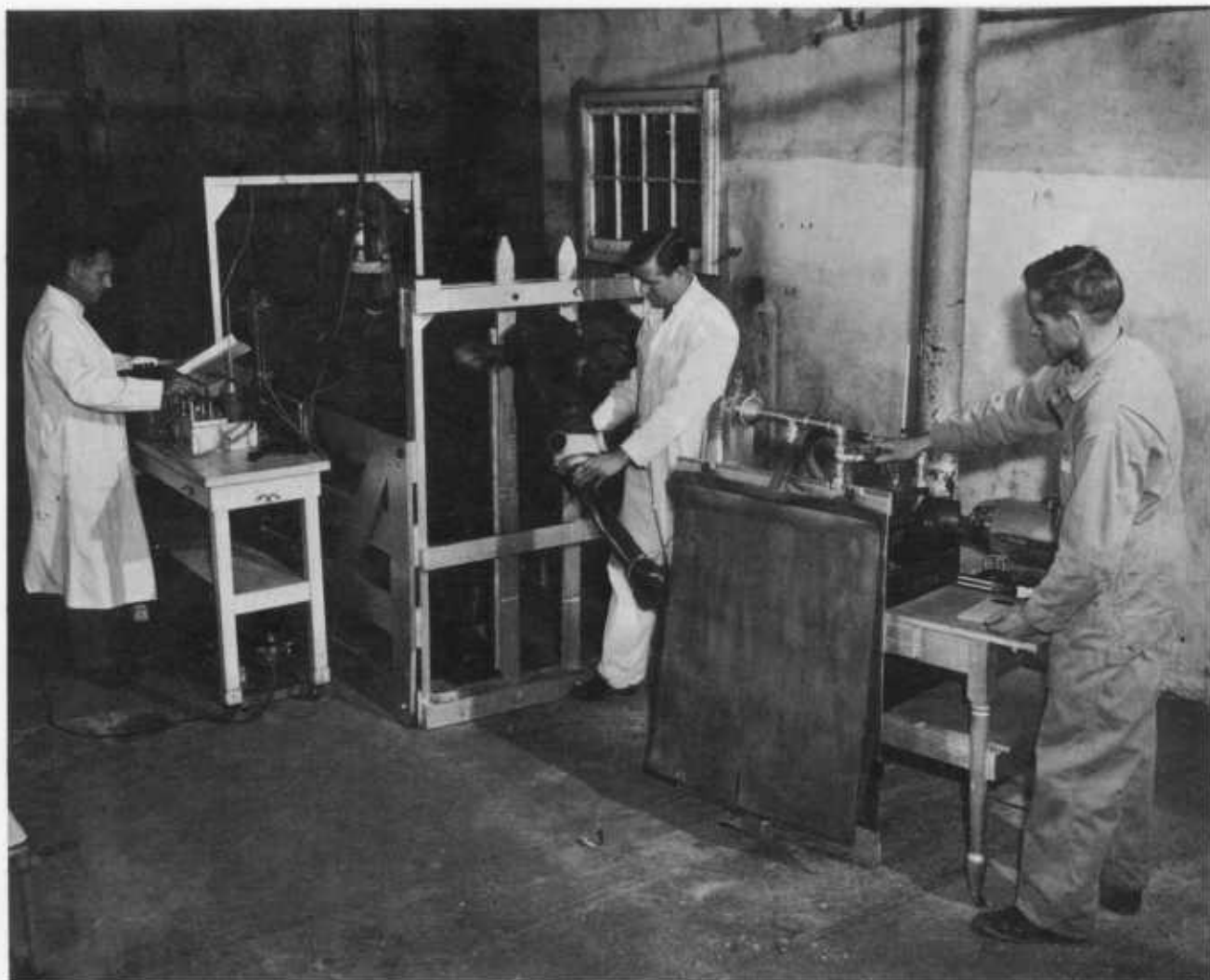
Scientists measuring respiration rate and volume of skin evaporation under hot conditions in the adaptability laboratory at the Center.
