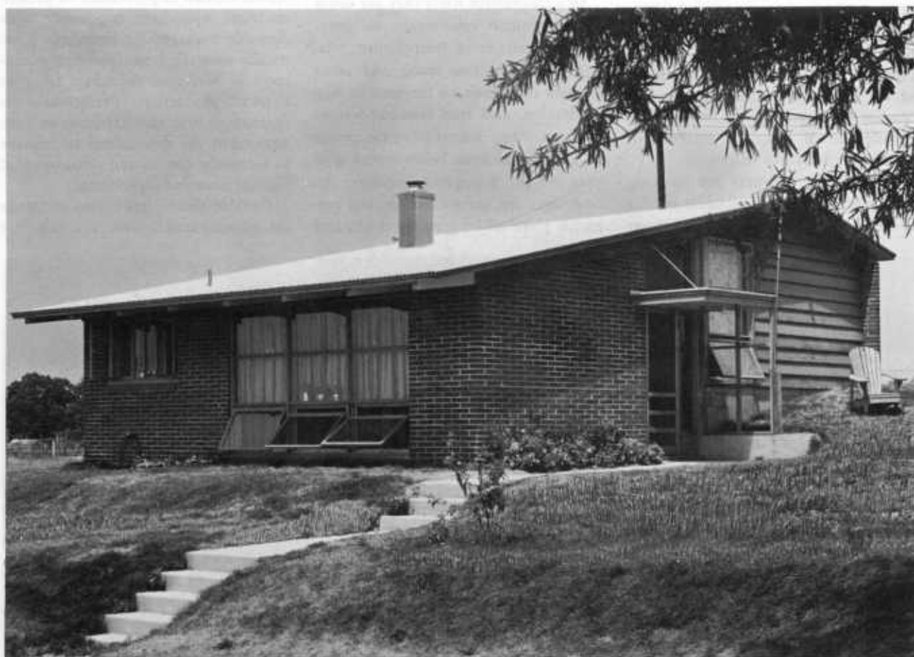
Split-level, expansible house with special large bricks for walls, plank-and-beam roof covered with corrugated aluminum, and a warm-air, perimeter-type heating system.
