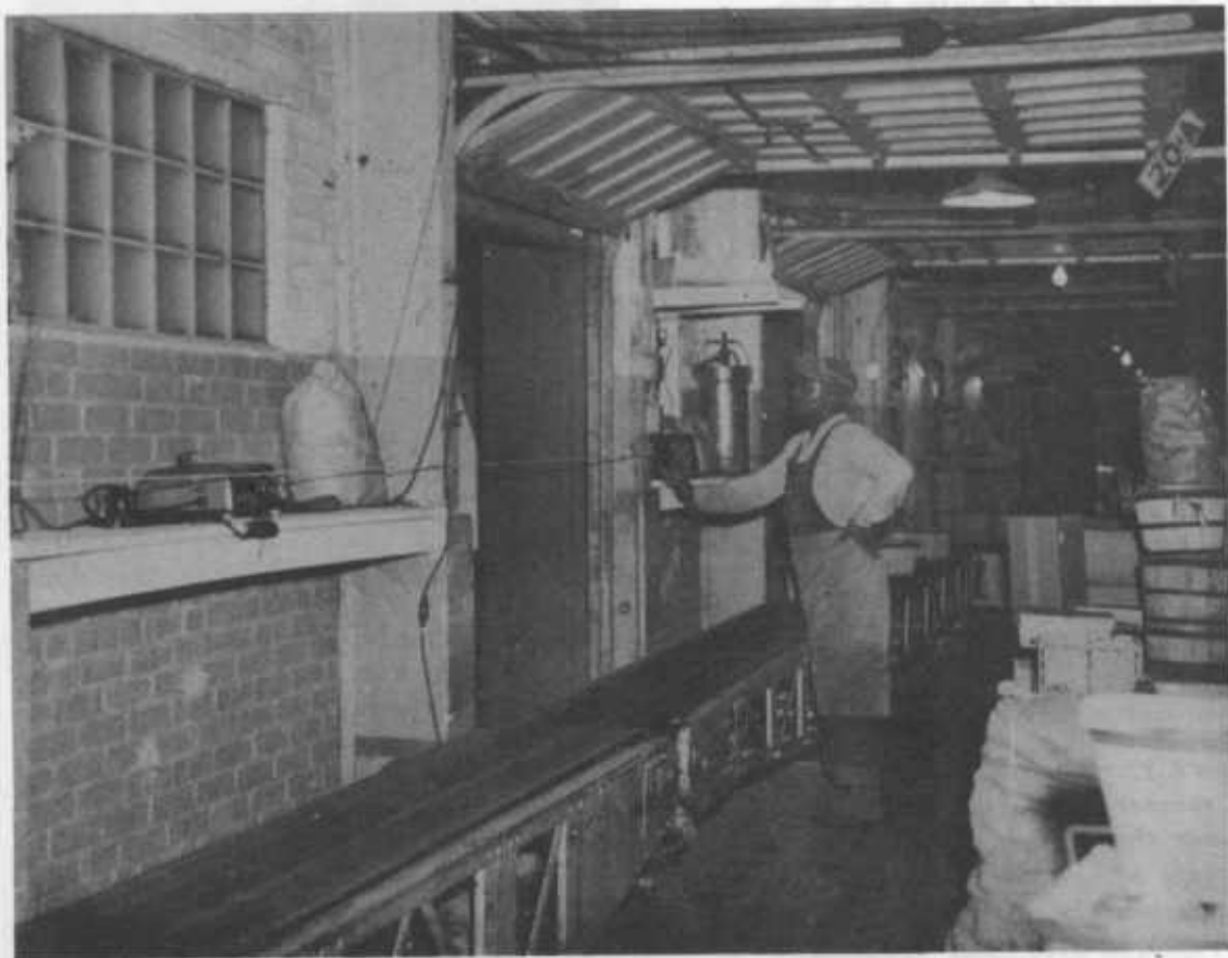
Figure 13.--Worker pulling cord which moves the arm on the micro-switch, thus completing the circuit to the transcriber and causing the items to be called over the loud-speaker.
