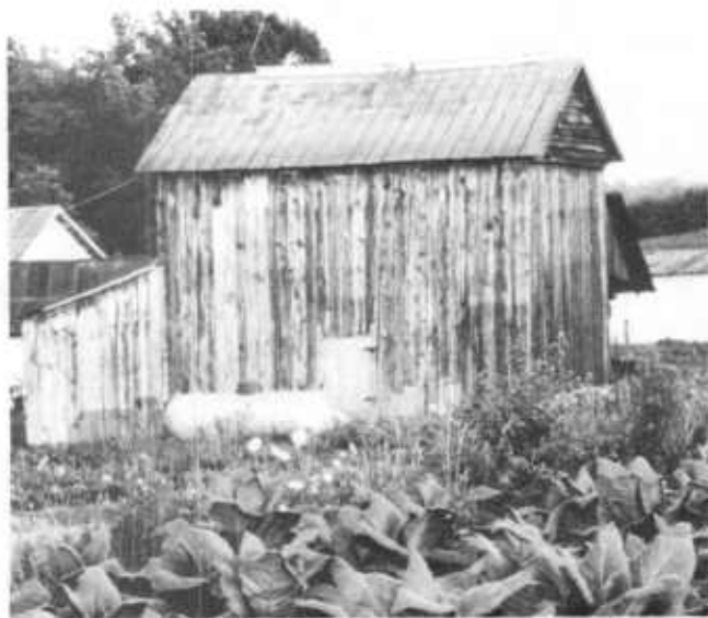
Traditional or conventional wooden flue-curing barn. These barns are being replaced by the more efficient bulk barns shown at right.
