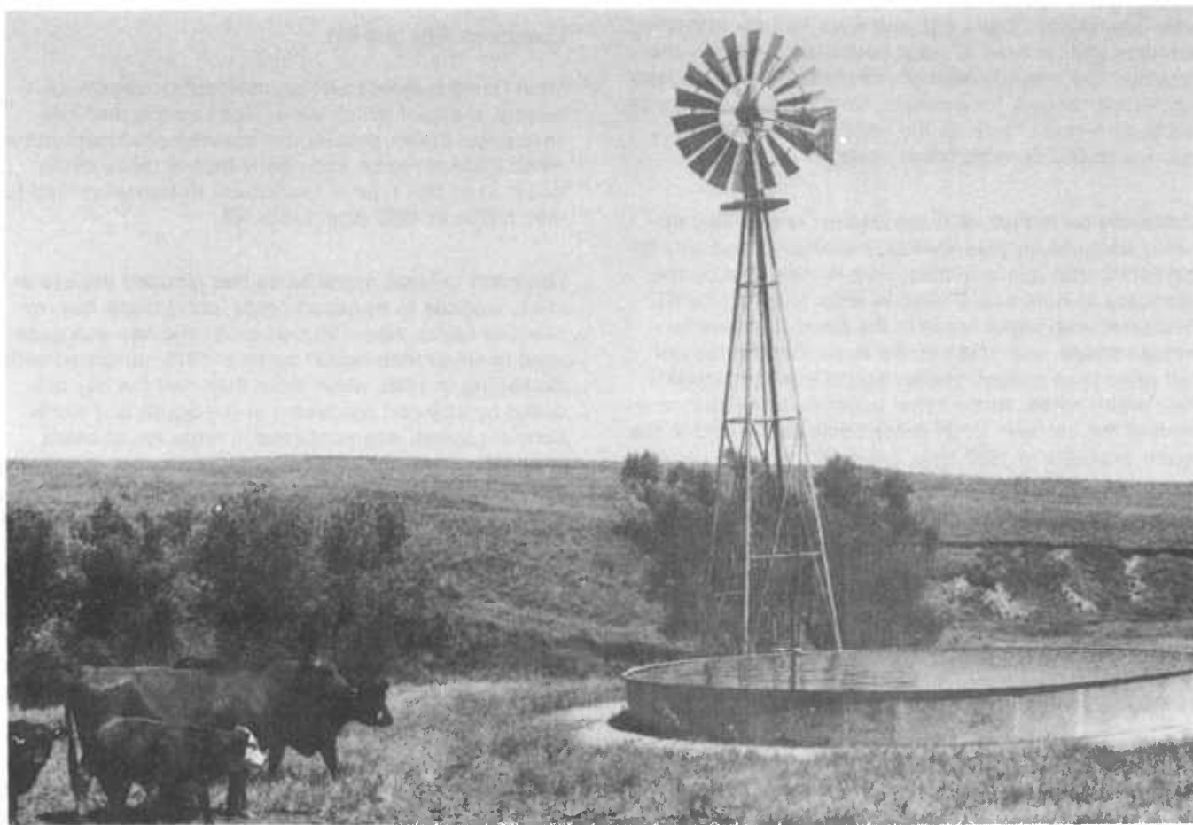
Windmills provide pumping power for nearly half of the wells used to supply livestock water in the Great Plains and West, where subsurface water must be provided in remote locations to permit effective grazing of large dryland range areas.
