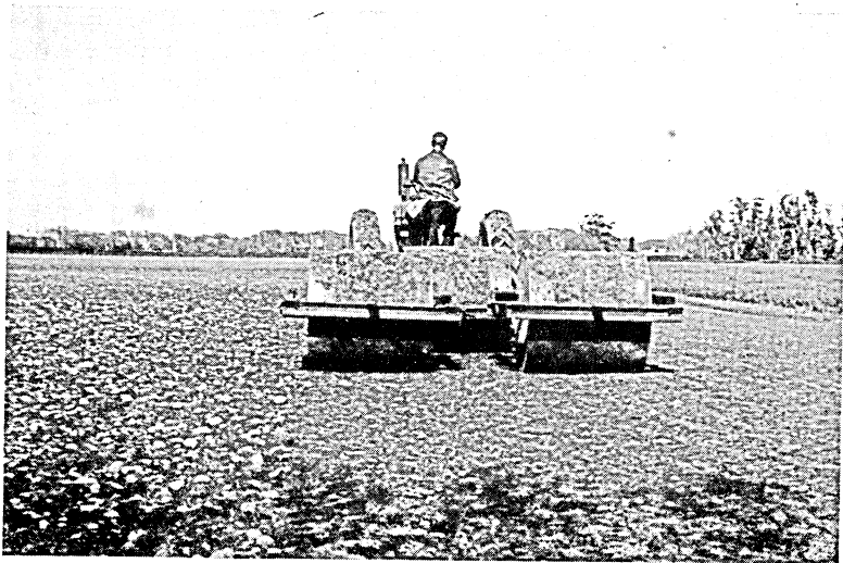
Seven-ton roller at work. Pad. 11.
