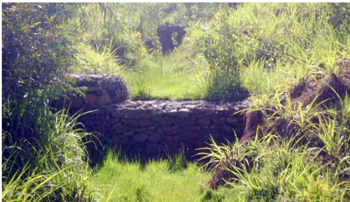
FIGURE 5. Gabion check dam supported with elephant grass in Alekit-wonz watershed, Amhara region.
