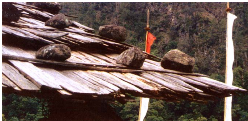
Wood shingles are among the many products the villagers make from local trees. Villagers use rocks to hold shingles in place during strong winds.
