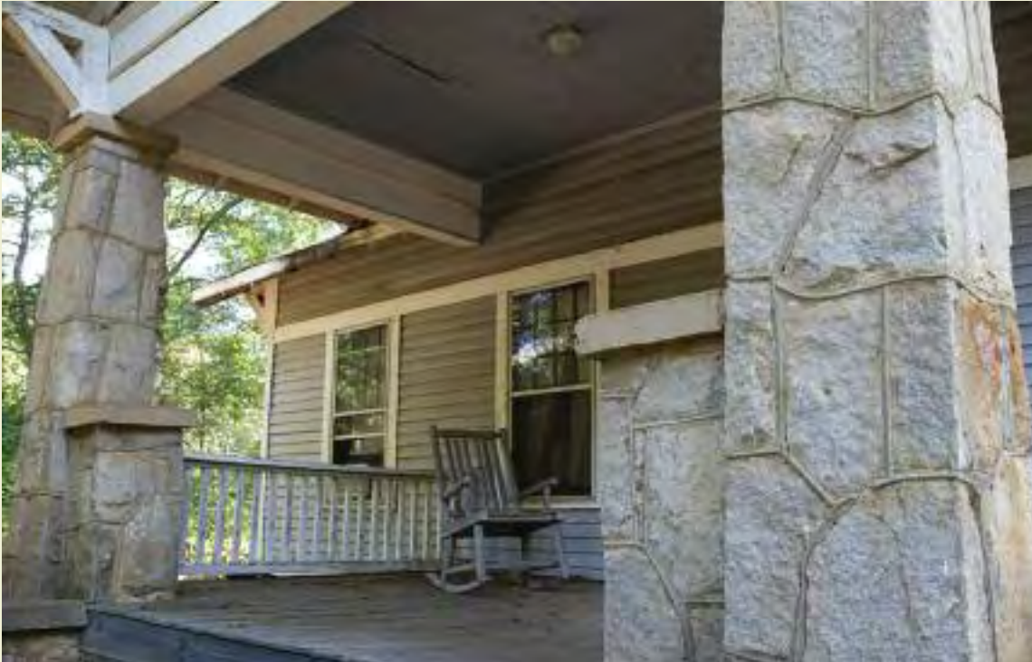
The stone for the columns of Maureen Richardson's home in Good Hope, Ga., was hauled by train from Stone Mountain in 1916. With help from Walton EMC's Operation Round Up, other parts of the home will get needed revitalization. Photo courtesy Walton EMC
