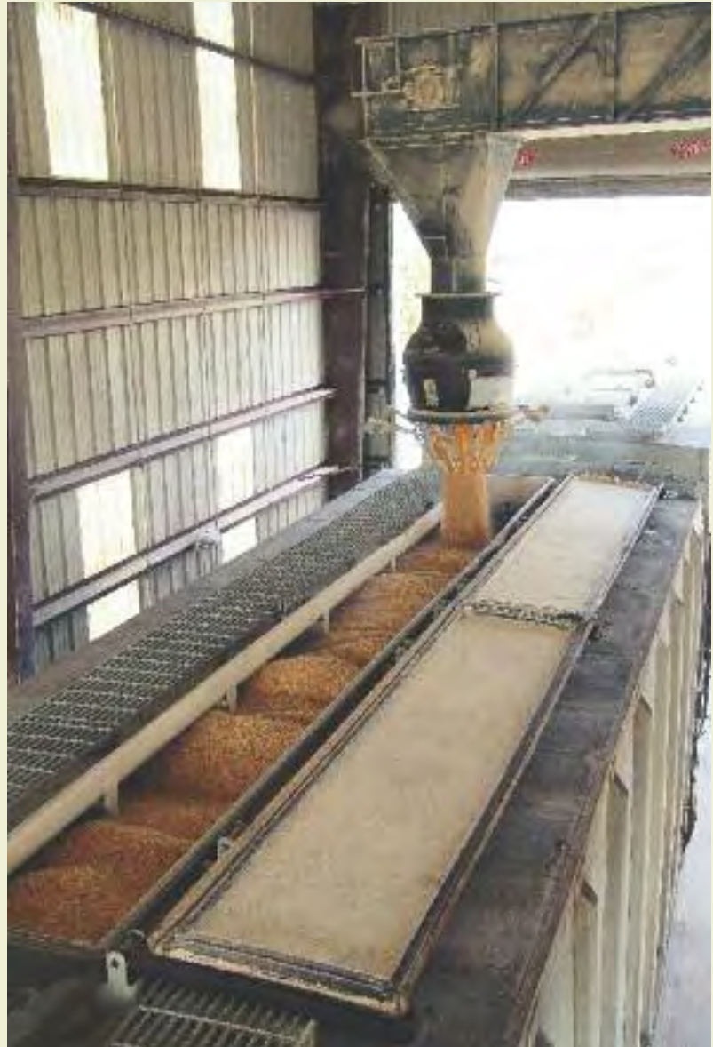
The co-op's rail facility at Linville, Va., has enough rail siding to store a 125-car train. It can unload 75 cars in 16 hours.
