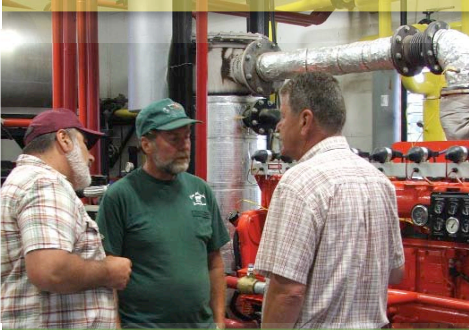
Vermont dairy producers Brian Rowell (center) and Bill Rowell (right) check on the on-farm generator that produces electricity from a manure-to-methane gas digester on their Green Mountain Dairy Farm. Photo courtesy University of Vermont Cooperative Extension
