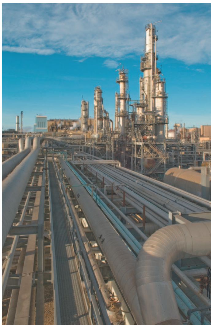
The Great Plains Synfuel plant, run by a Basin Electric subsidiary, converts dirty, low-quality lignite coal into clean-burning natural gas. The carbon dioxide generated by the conversion is recovered and injected into Canadian oil fields, forcing out petroleum that would otherwise be inaccessible.
