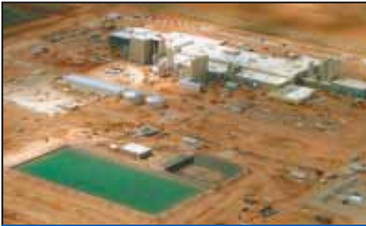
Work is progressing on the new DFA /Glanbia PLC cheese plant in New Mexico .
